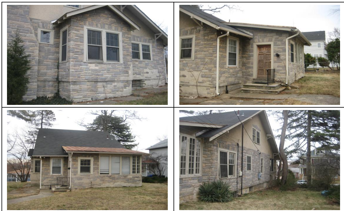
Figure 8: Building C – Exterior
