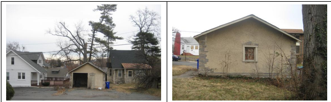
Figure 7: Building B - Exterior
