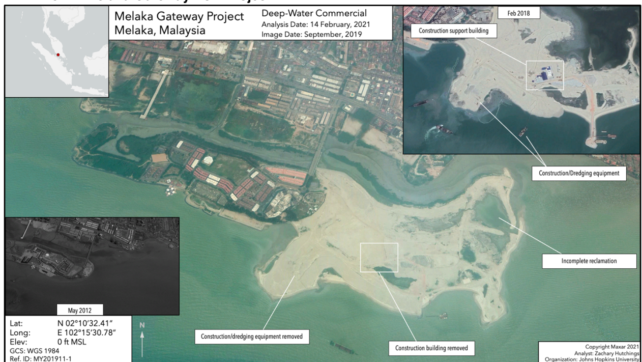
Image 5.1.2: Melaka Gateway Port Project Graphic
