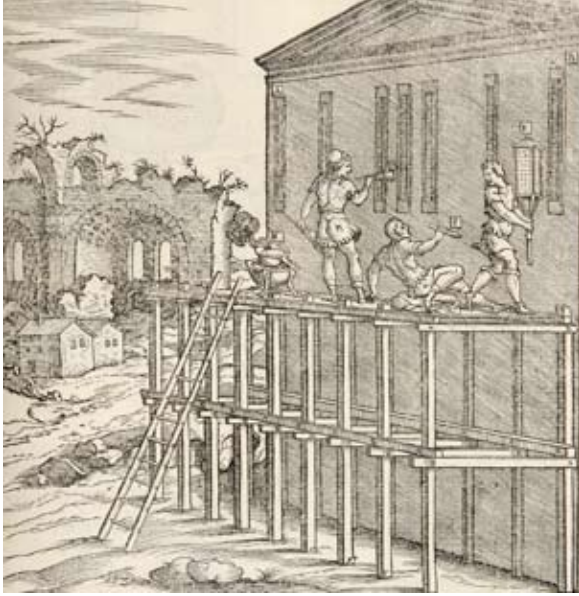
Masons laying brick
