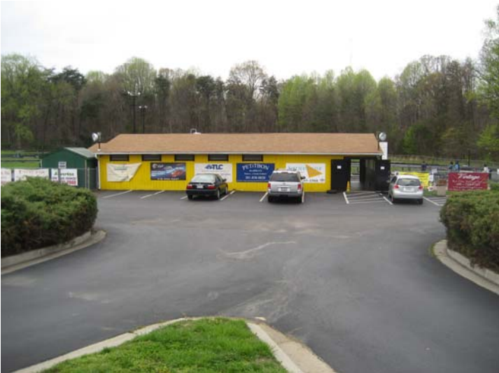
EXISTING STRUCTURE ON SITE (WEST VIEW)
