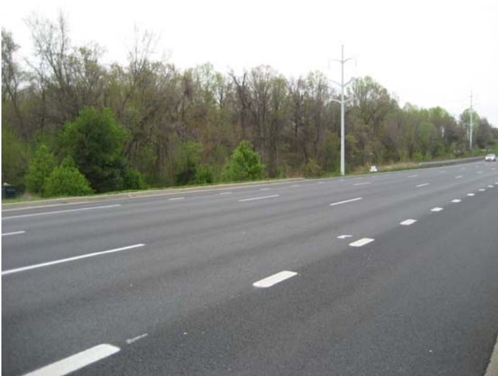
LAND NORTH OF SITE (UTILITY EASEMENT)
