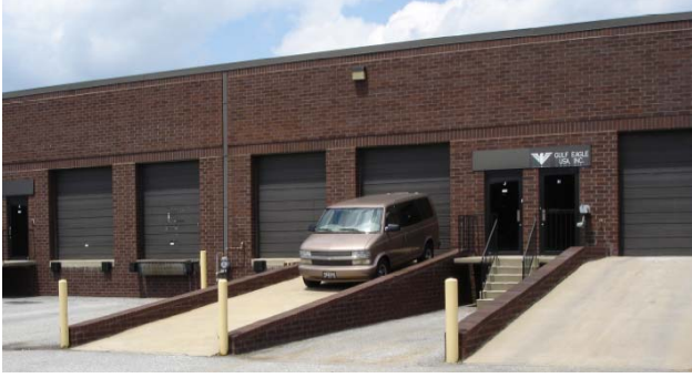
Truck Court - Dock & Ramp Loading
