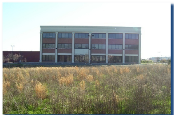
View Looking South to Madison Square Office Building from 300'± into Property
