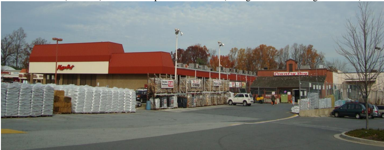
Existing use on Parcel I (Country Boy) in the subject site
