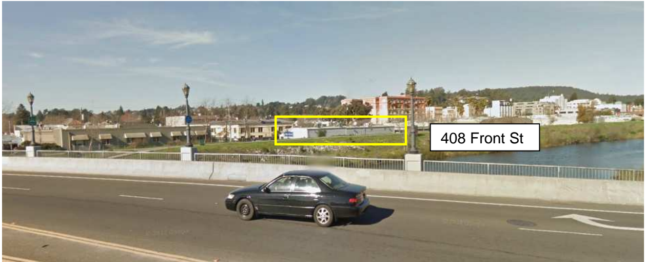
Figure 21: View of 408 Front St from Laurel St Bridge (Source: Google Street View)
