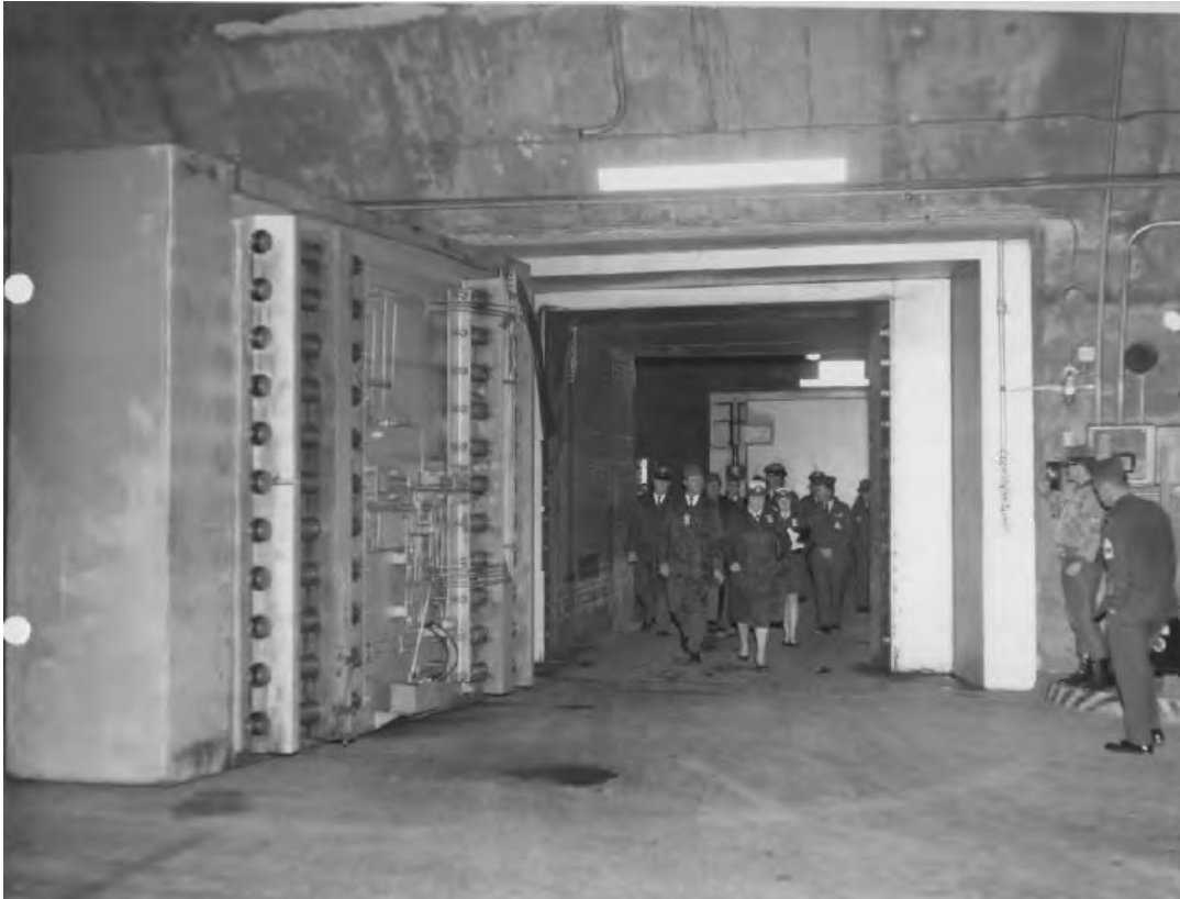
Figure 24. Massive blast doors could be opened within 30 seconds. Source: Marian Talmadge and Iris Gilmore, NORAD: The North American Air Defense Command (New York, NY: Dodd, Mead & Company, 1967).
