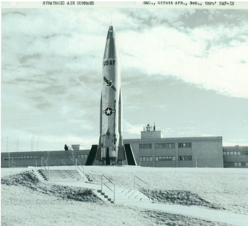
Figure 15. View of Building 500, SAC headquarters at Offutt Air Force Base. Source: USAF.
