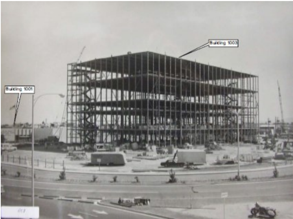
Figure 33. The Blue Cube, Building 1003, under construction in 1968. Original photograph source: Onizuka AFS. Annotated by Jennings and Rachleff.
