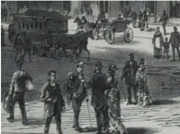
Figure 6. Detail from a drawing of the Central Hotel in Berlin (op. cit., fig. 4).
