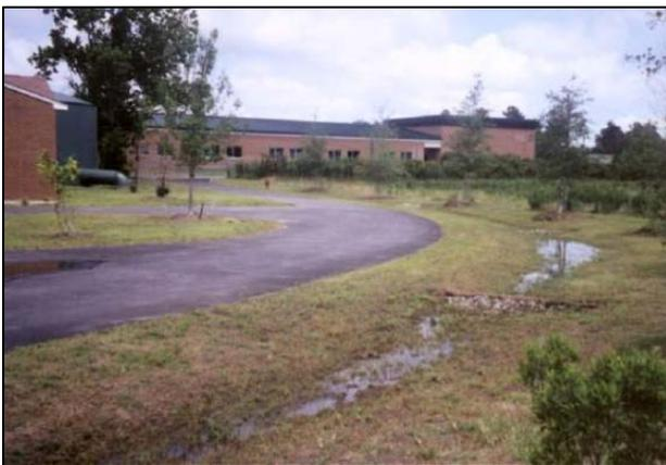
Grass channels can provide a modest amount of runoff filtering and volume attenuation within the stormwater conveyance system resulting in the delivery of less runoff and pollutants than a traditional system of curb and gutter. The performance of grass channels will vary depending on the underlying soil permeability
