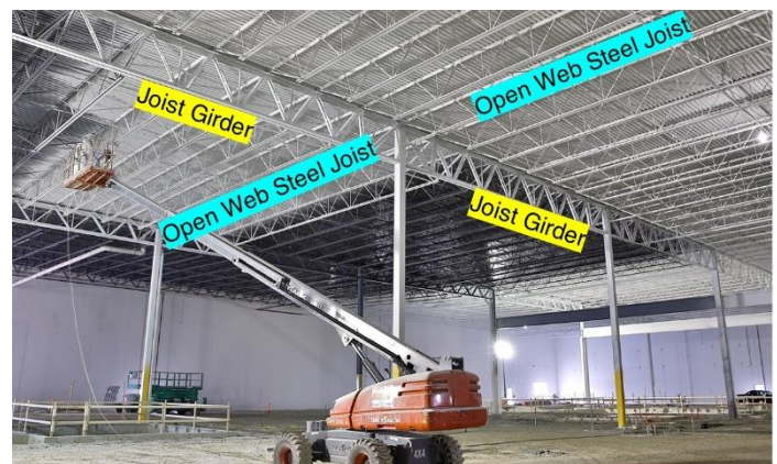
Figure 1: Photographic view of metal industrial buildings Taken from www.newmill.com
