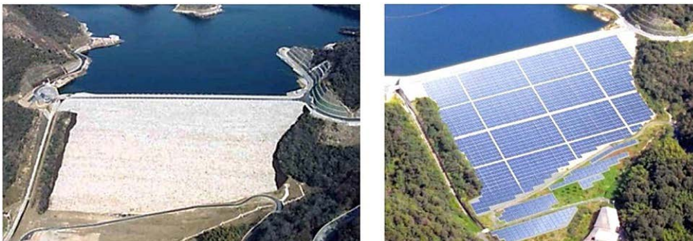
Figure 8: Japanese PV installation on dam face (Kougias et al, 2015)
